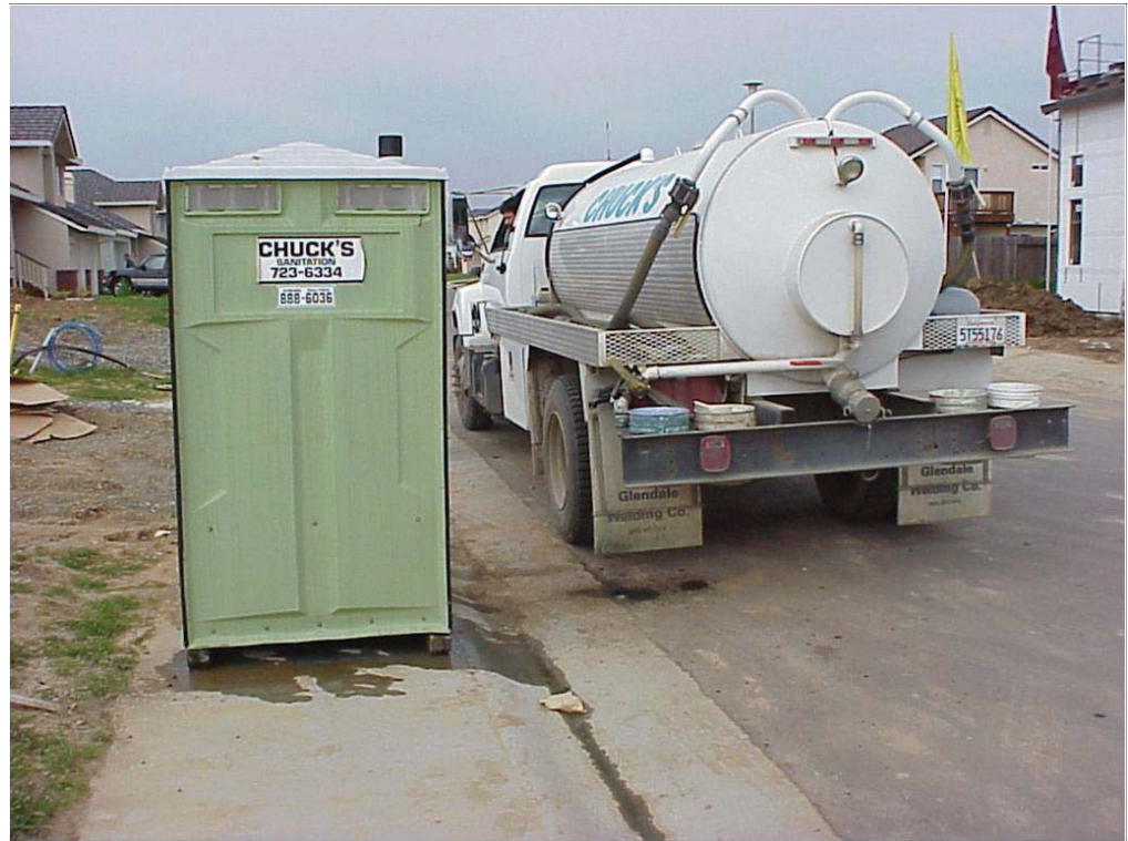
Improperly managed and leaking temporary sanitation facility.
